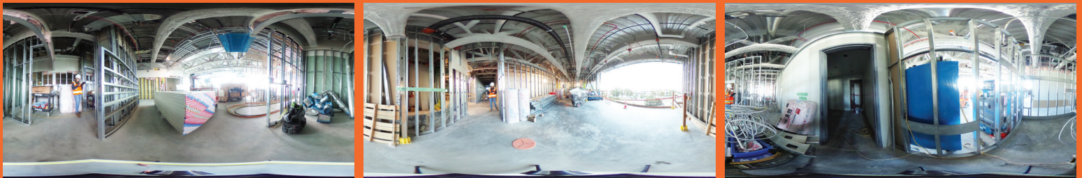
Captured 360 Site Photos Using StructionSite
